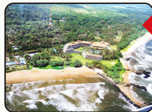
Development activities in accordance with coast conservation permits enhance the beauty of the coastal environment
