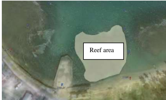
Figure 4-16: PPD2-RL- Area west of the jetty studied in addition to the systematic samples
