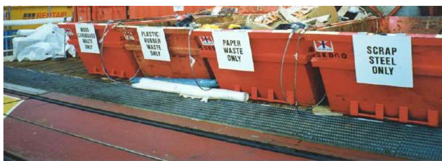
Figure 4: Large dumpsters to store construction waste
