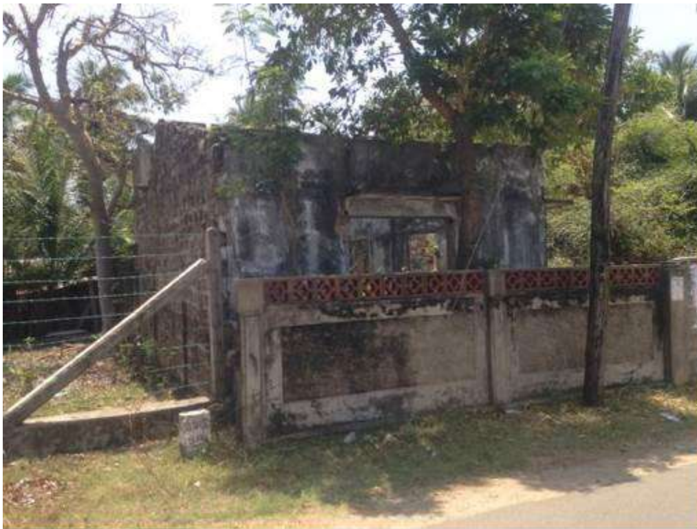
Fig. 12. Abandoned homesteads with vegetation including Morinda coreia
