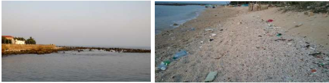
Figure 3-5 Nature of the shore; To the east is a revetment and to the west sandy beaches
