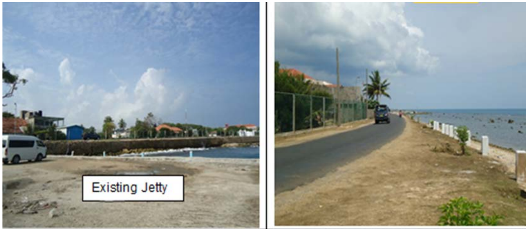
1. Western Site of project area
