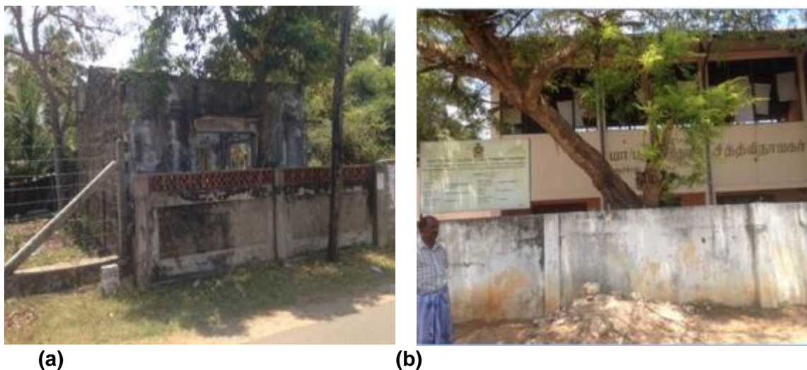
Figure 4-31: Abandoned houses and Sitthy Vinayagar School within the PIA of the PPFHDP.
