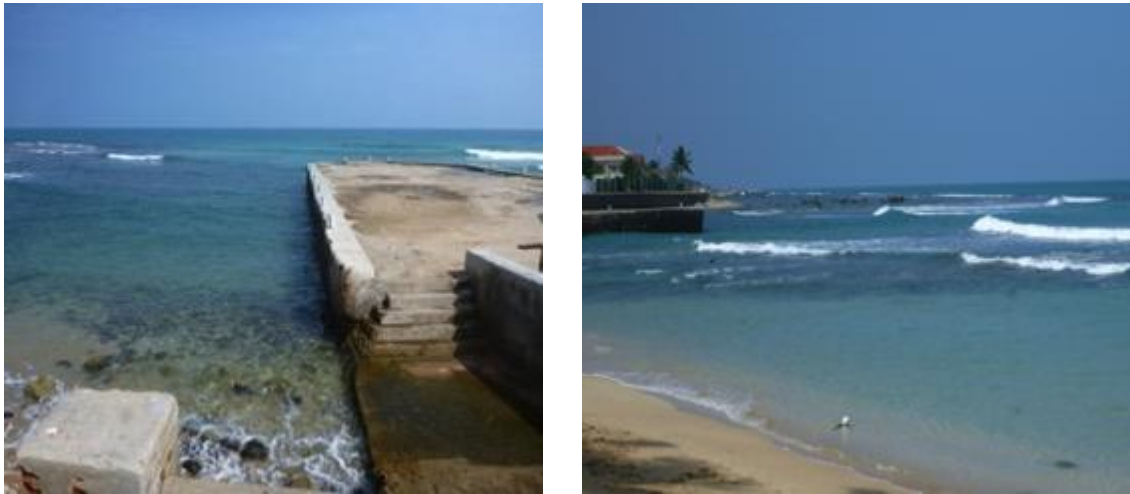
Figure 1-4: Point Pedro Existing dock facility.
