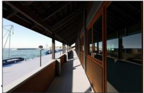
Administration Building Front Verandah 1 st Floor
