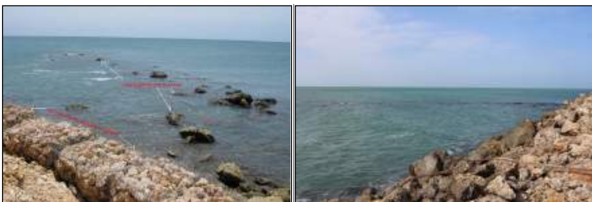
Figure 2.7: Condition of the Northern Arm
