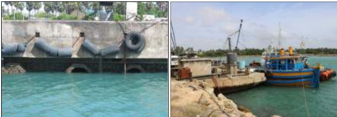
Figure 2.5: Condition of the Existing Pier No. 1
