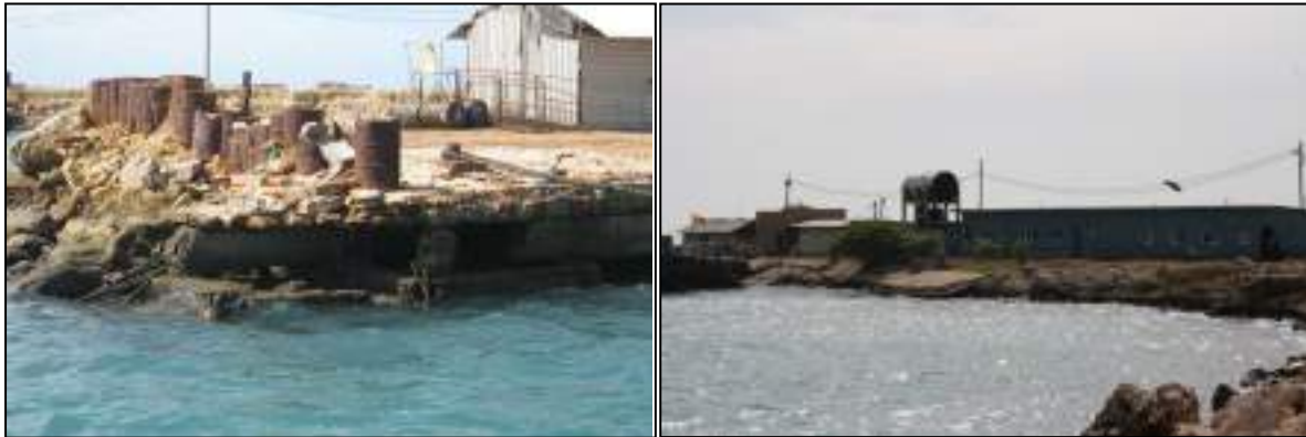
Figure 2.6: Condition of the Existing Pier No. 2
