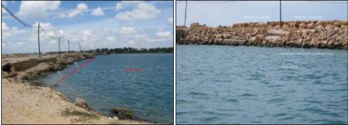
Figure 2.4: Condition of the Existing Breakwater
